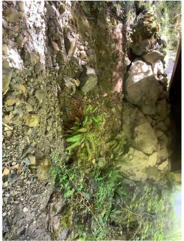
Right Bank Abutment when facing downstream
